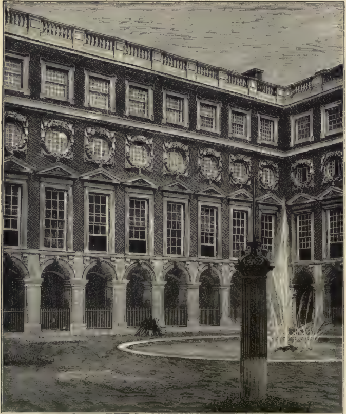
Part of Hampton Court ; built for William III. by Sir Christopher Wren.
